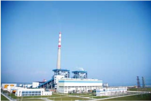
Beihai power plant
