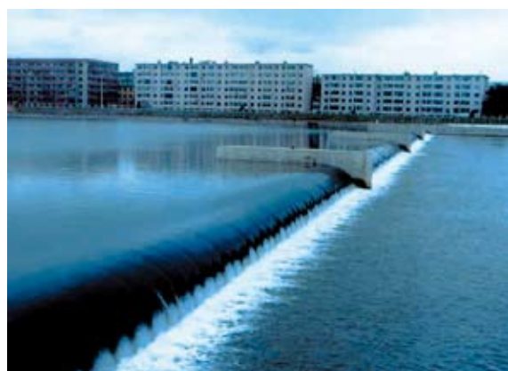
Yanji Rubber Dam Project
