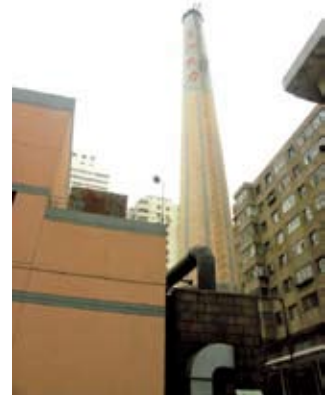
Lanzhou Thermo-electric Plant
