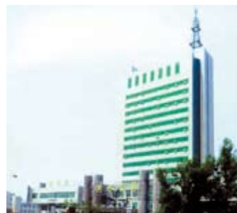
Daqing Water Works
