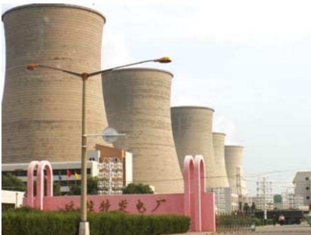
Baotou Dalate power plant
