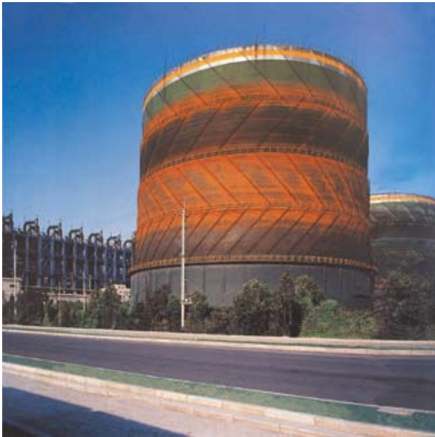
Shanghai Cokeoven Plant
