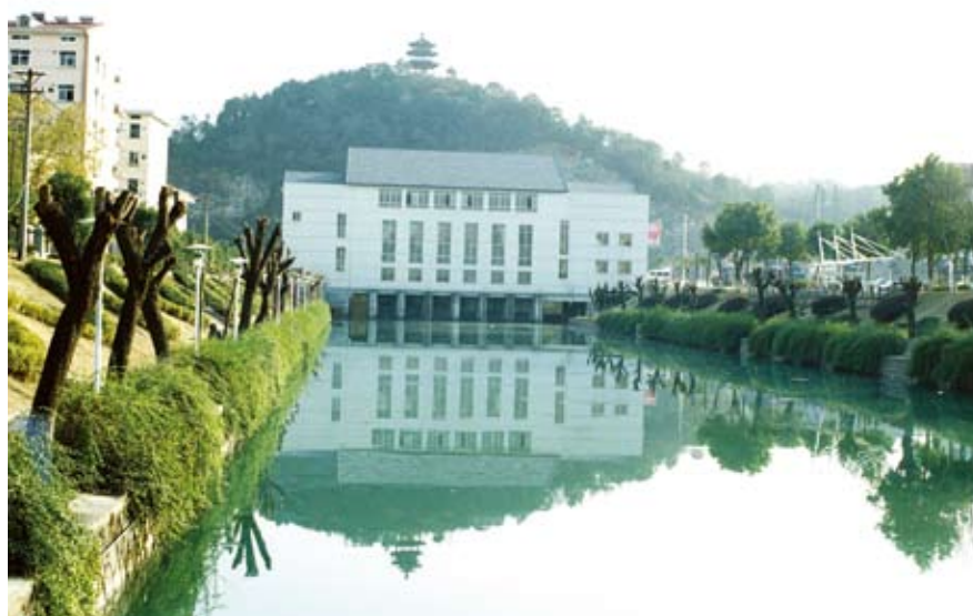
Changshan water conservancy
