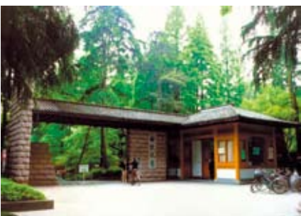
Hangzhou Quyanfenghe Pumping Station
