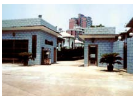
The Second Sewage Treatment Works, Changsha
